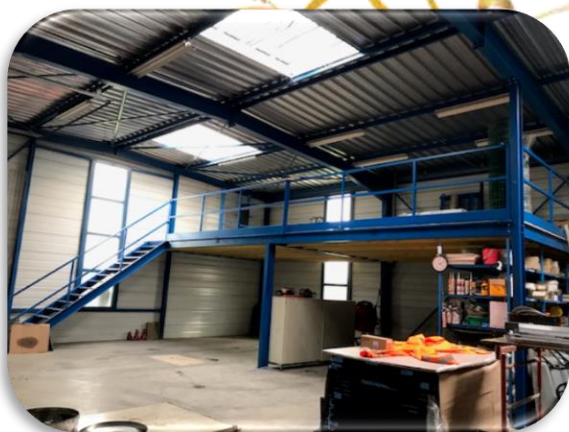
Installation mezzanine - Atelier municipal
